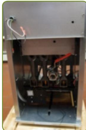
**7E:** Locate the white and black wires from the power harness and connect them to the like color wires of the transformer on the header.
