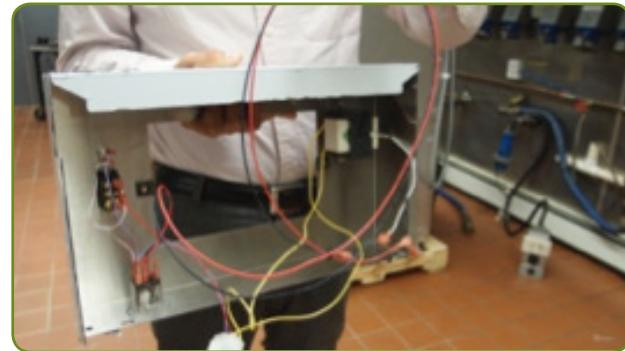
**8A:** Locate the red and black wires from the gas valve cut from the T-stat. Strip and crimp the male fastens on each.
