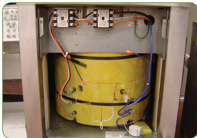
BEFORE INTERFACE HARNESS INSTALLATION
