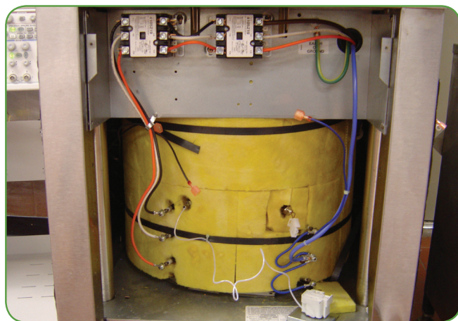
BEFORE INTERFACE HARNESS INSTALLATION
